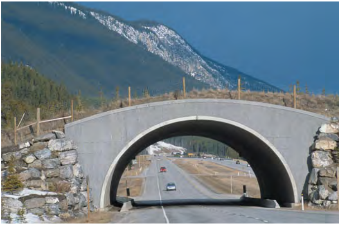
▲ Figure 56.18 An artificial corridor. This bridge in Banff National Park, Canada, helps animals cross a human-created barrier.
