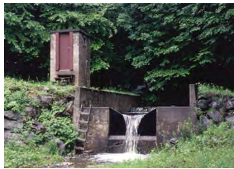
(a) Concrete dams and weirs built across streams at the bottom of watersheds enabled researchers to monitor the outflow of water and nutrients from the ecosystem.
